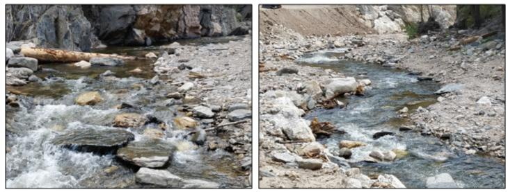
Figure 29-Deep constructed pools alongside bedrock with log enhancement & expanded floodplain
