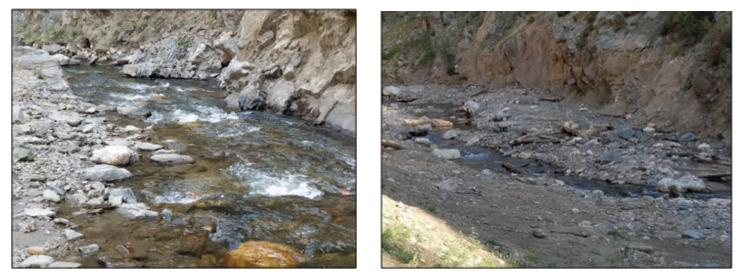
Figure 16-Riffle-pool sequencing and expanded floodplain bench above bridge on left and downstream of bridge on right
