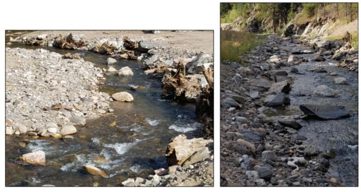
Figure 23-Root wad revetment at horseshoe bend & channel downstream of Bridge 8
