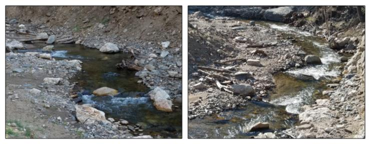
Figure 17-Expanded floodplain capacity upstream and downstream of Bridge 5
