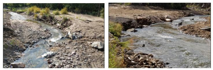
*Figure 26-Channel meandering, root wad revetment and boulder clusters downstream of Bridge 11*
