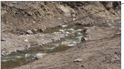
*Figure 11. Floodplain benching, riffle-pool sequencing, boulder clusters and habitat wood in the beginning of a backwater pool (river left top).*
