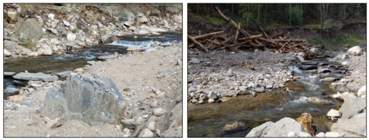
Figure 28-Strategic rock placement for riffle-pool morphology & log jam on expanded floodplain
