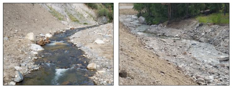
Figure 30-Expanded floodplain benches, root wad installation, meandering channel, riffle-pool sequencing
