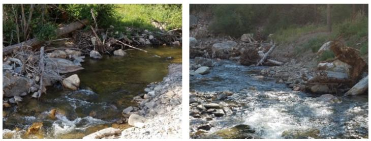
Figure 20-Pool habitat upstream of tributary & root wad revetments downstream
