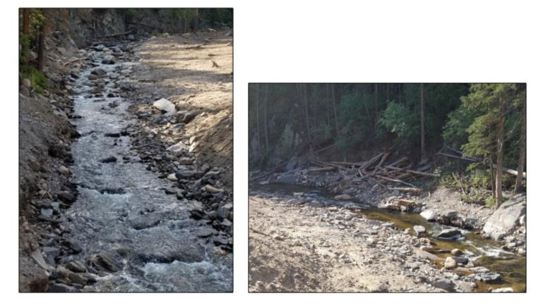
Figure 22-Expanded floodplains, boulder clusters, constructed large woody debris up and downstream of Bridge 7
