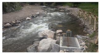
Figure 9-Fish friendly irrigation diversion
