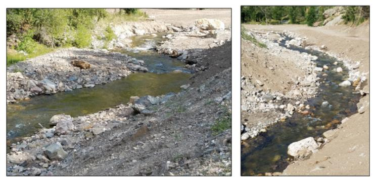
Figure 25-Meandering riffle-pool complex using primarily boulders at Ballard site
