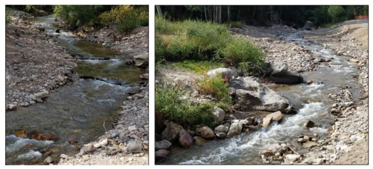
Figure 27-Floodplain grading and boulder placement at Whiteside
