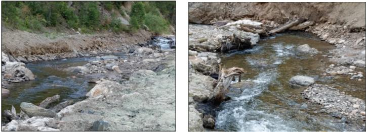
Figure 15-constructed step-pools on left and root wad revetment with habitat wood on right upstream of bridge
