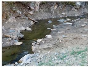
*Figure 5. A constructed low-flow channel, point bar, installed habitat wood, and increased channel sinuosity downstream of bridge 3*
